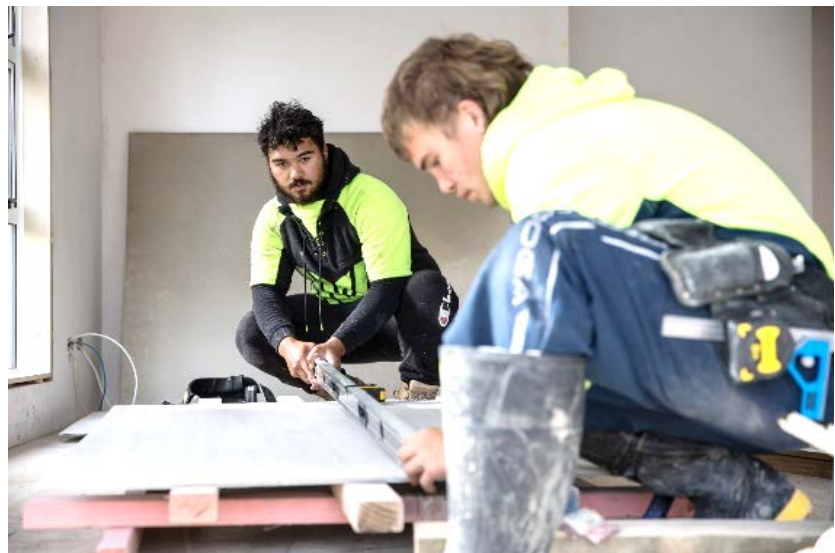
Figure 19. Qualified builder and Senior apprentice at work.
