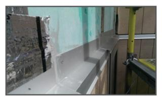
Scribe measurements before cutting. Dry fit and re-cut if needed, then silicon edges/joins so no water can get into building. Tape along top joins, along top flashings and onto rab board.
