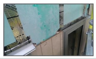
Once the window was installed, we used a level to run across to the other window to see if it was level to make the flashing easier to put on.
