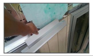
Then I measured the flashing in between the windows, siliconing top of shadow clad before attaching the flashing to the cladding.
