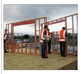
We started on the blocks. We needed 12 in all and we cut them roughly to 200mm each. We put four nails in each of the middle ones for the partition, which is tricky since the stud gets in the way. We couldn't nail on an angle since these ones were 90mm wide and 45mm deep unlike the other eight which were the opposite way round. We had to nail on a slight angle while trying not to hit the stud in front.
