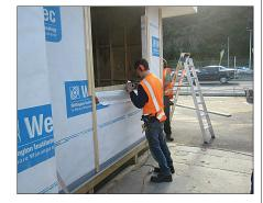
against the face of the internal wall to ensure the window was in place. We checked the allowance for the 10mm internal gib linings. We tacked a 75mm jolt head galvanised nail to the side jamb at approx. 70mm from the corner, two to each side, one at the top and one at the bottom. For a larger window intermediate nailing is required. After making sure that the window was plumb, packed and sat centrally within its opening, the nails were then placed and punched in.
