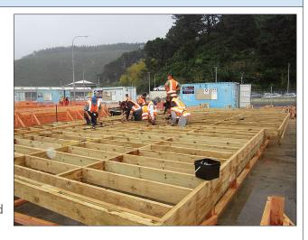
We cut the four joists (using the drop saw) and nailed them in. We had to trim a few down so they fit in between the piles.
