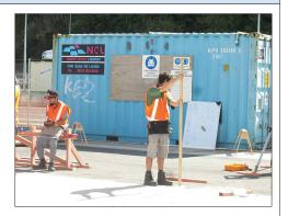
The datum was three sites over. We marked the 140mm mark the dumpy was reading onto the staff.
